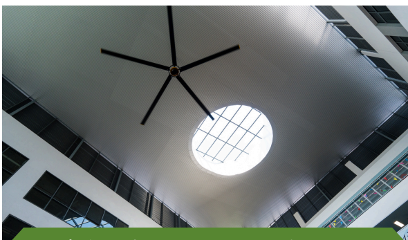
High Volume Low Speed (HVLS) fans for air circulation
