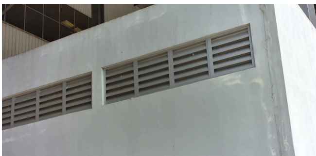
Natural ventilation louvers for improved airflow
