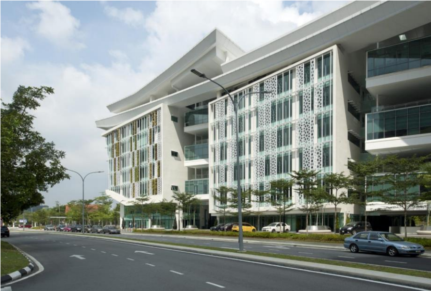
Partial facade views of office blocks and floating meeting rooms with DGU curtain walls and islamic motive sunscreen
