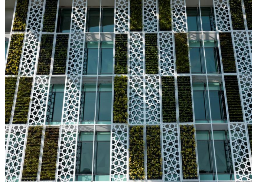
Close-up facade views of office blocks with DGU curtain walls and islamic motive sunscreen
